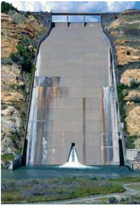
The spillway at the Navajo Dam. Notice the bottom release that keeps the water at a constant temperature, creating an amazing tailwater fishery.
